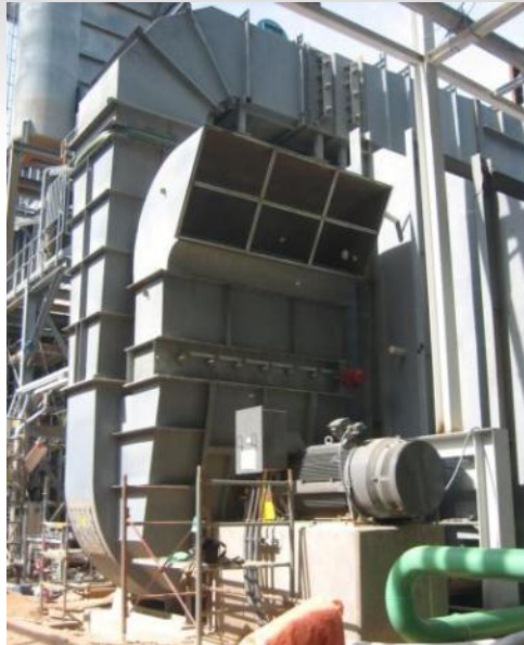
DIAF 691-3095-100 SWSI, Airfoil Bladed Draft Fan, Arrangement 3A
