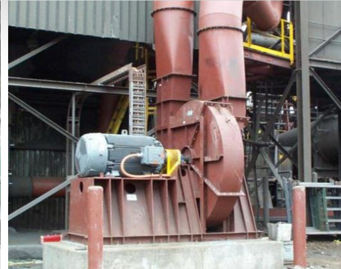
DRBO 1540-85% SR.20, Radial Bladed Exhaust Fan, Arrangement 7B
