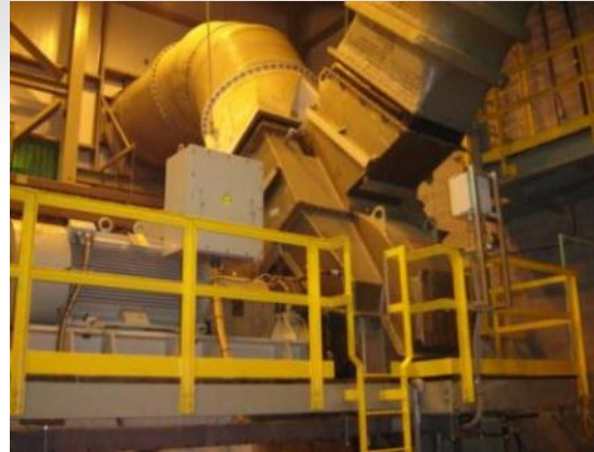
DSTA 650 Sr. 3057 Cl. 35K DWDI, Backward Curved, Arr't 3D
