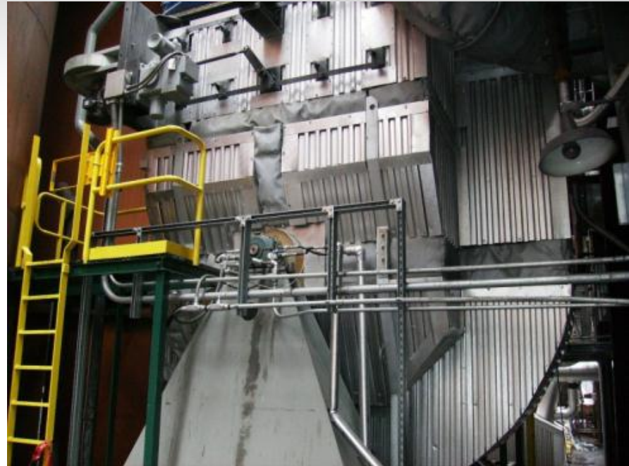
DRBS 2316 SR.47 SWSI, Radial Bladed Draft Fan, Arr't 7B
