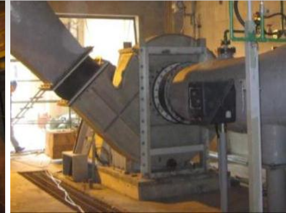
DRBS 1148 Sr. 42 SWSI, Radial Bladed Fan, Arr't 8A
